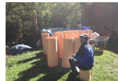
Rosberg H. T., a water filter technician for DESEA, is preparing biosand filters for installation in Lamay, Peru. Photo taken in 2014 by Green Empowerment's Bryan Ferry.
