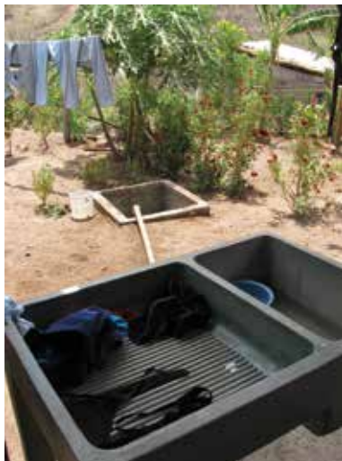
A greywater system reuses dishwater by piping it directly to patio gardens, El Jocote, Nicaragua, 2013.
